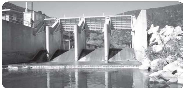
Looking upstream at the Robles Diversion Dam on the Ventura River. A new fish ladder will reestablish upstream passage for the first time since 1958.
