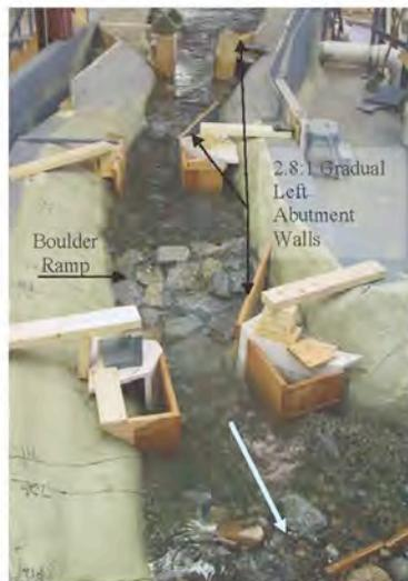
1) View looking upstream at the Alternative 4 intakes operating at 900 cfs. Note the boulder ramps downstream of each intake and the addition of a more gradual alignment to the left side upstream abutment walls. (DMG\_6773)
