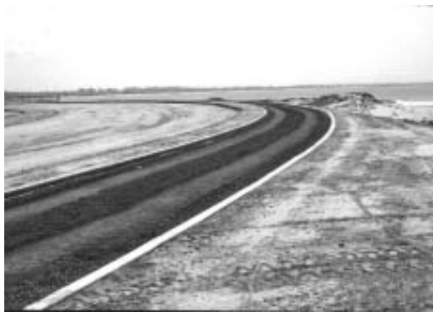
Figure 2: Construction of the Surfers Point parking lot and bike path, 1989.
