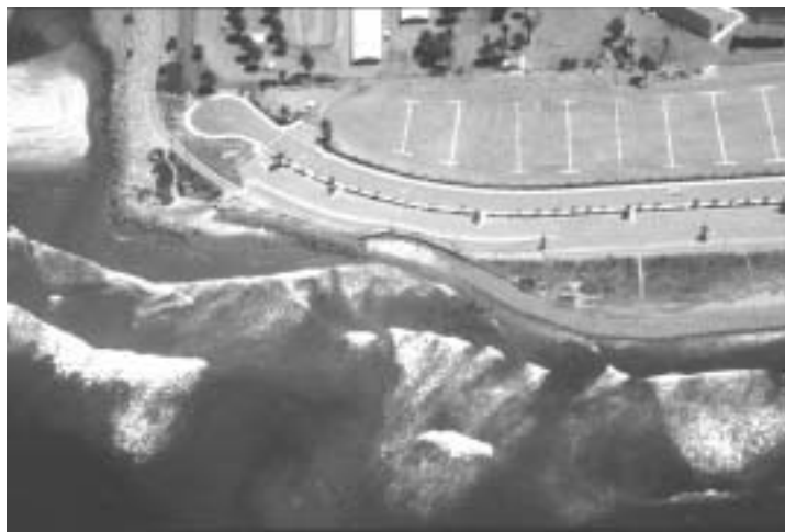
Figure 3: Parking lot and bike path near the mouth of the Ventura River, 1995.
